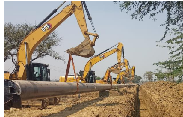
Slurry Pipeline laying in Odisha
